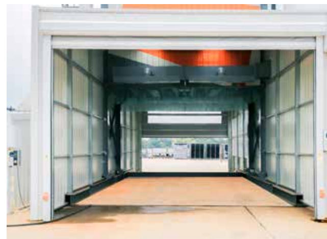
● 卸料系统：主楼接料通道封闭效果图 Effect Picture of Enclosed Main Tower Receiving Channel for Discharging System
